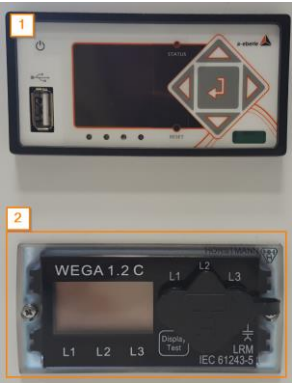
Figure 20: Installation example EOR-3D compact and voltage tab of WEGA 1.2C
