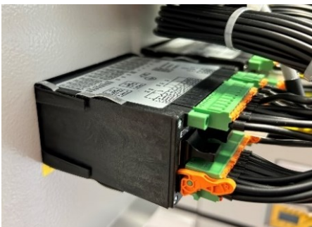
EOR-3DS in control panel cut-out
